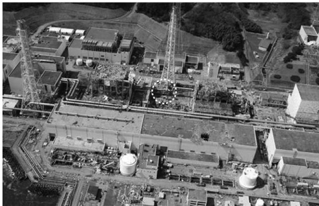
Figure 17 Damaged R/Bs of Units 4 and 3 and T-shape connected vent pipe at the lower end of stack. (Photo: Air Photo Service)
